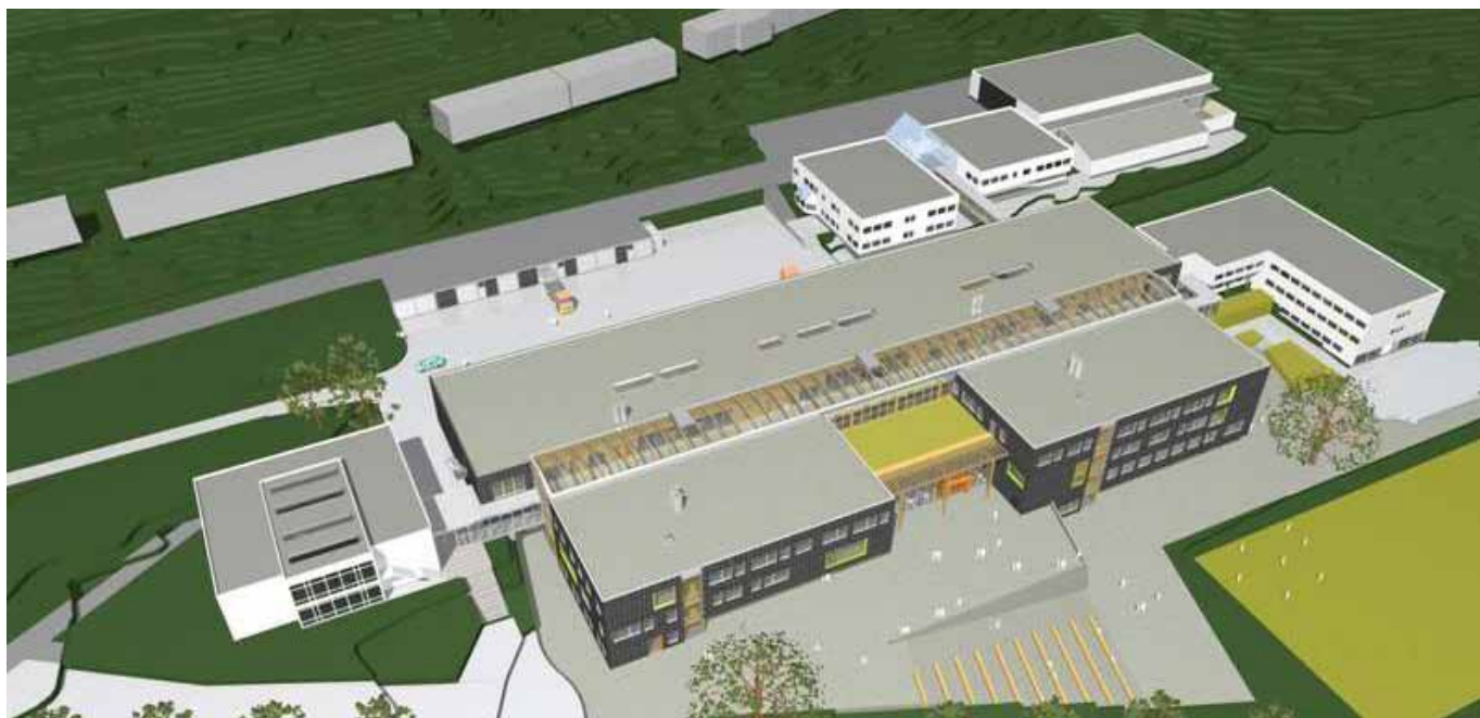
Betonmast: Romsdal Videregående Skole
